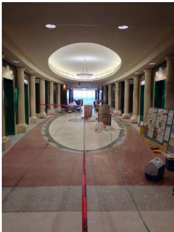
Work on the 16th floor is almost done.
